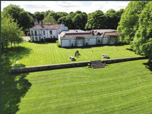
Entrances complete with porticos leading to formal lawned terraces with a Ha-Ha wall
